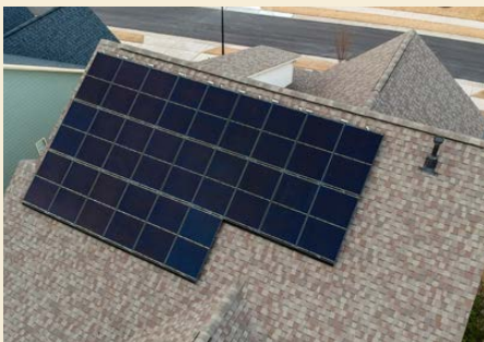
Is free from obstructions like vents and dormers
